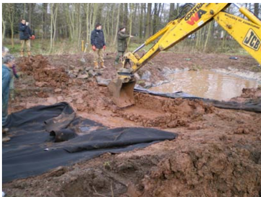
Constructing the Dividing Bank
